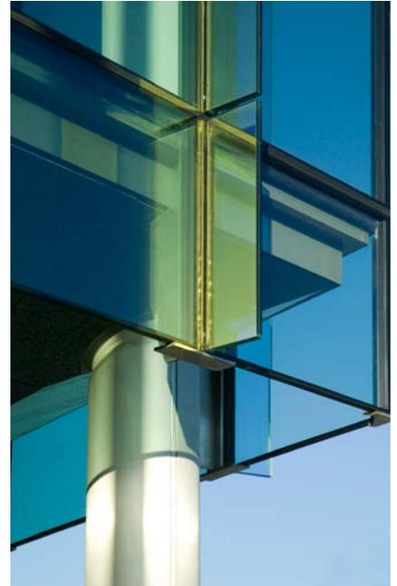
NARIMA® Color Effects Glass is available in standard thicknesses of 6 mm with a float glass base. It is also available using extra clear low-iron float glass and RIVULETTA® structured glass on request. 4 mm, 5 mm, 6 mm, 8 mm, 10 mm and 12 mm thickness also available on request.
