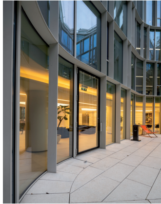
pic_02.tif: The round shape of the panes is easy to retrace on the floor covering.
