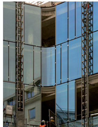
pic_05.tif: E30 was required from the 1st floor upwards – ISO PYRAN® G even achieved E60 in the test.
