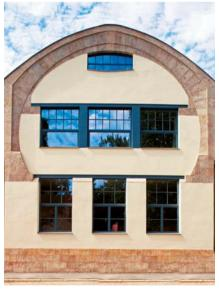
SCHOTT is not only capable of manufacturing modern glass, but can also manufacture drawn glass using the traditional Fourcault process. The restoration glasses RESTOVER® and TIKANA® feature the irregular, lively looking structure that is characteristic of historic window glass. This is achieved by manipulating during the production process.
