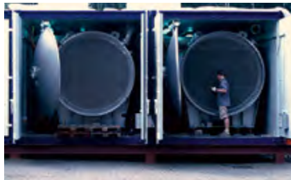
The ozone generators are installed in large-capacity containers.
