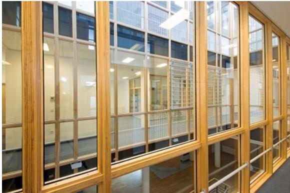
PYRANOVA® from SCHOTT is a reliable, high specification specialty glass for fire-resistant glazing combining full insulation with fire integrity and impact protection. Photo: SCHOTT.
