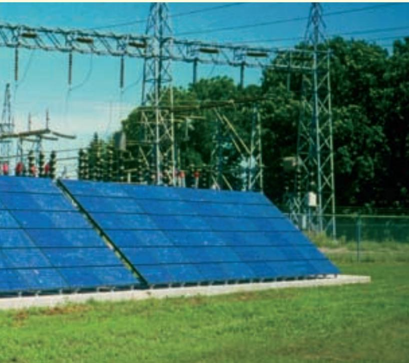
*The US General Services Administration in Suitland, Maryland operates a 100 kW thin film pilot unit. In comparison with conventional photovoltaic systems equipped with silicon wafers, here glass substrates coated with thin films are used.*
