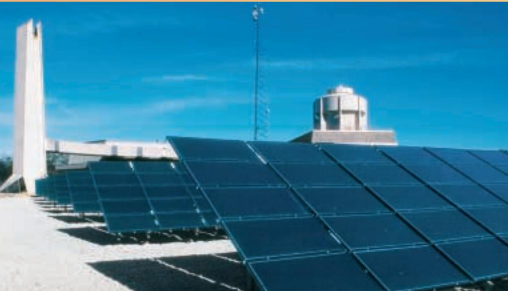
*A grid-connected photovoltaic array at Alliant Energy in Winnebago, Minnesota. It can be used to bridge any supply shortfalls at peak times.*
