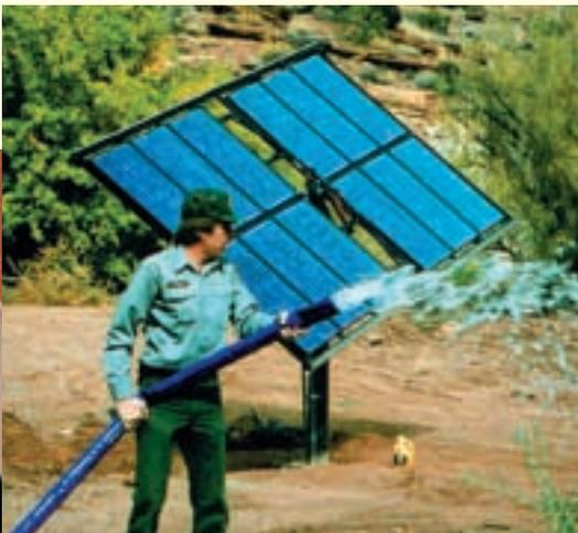
*An environmentally friendly alternative to diesel generators: The Capitol Reef National Park in Utah uses photovoltaic modules to pump water from deep below ground.*
