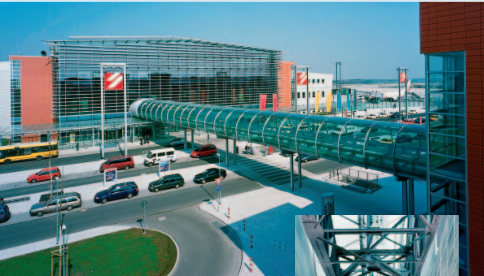
The view from the street is dominated by the prominent skywalk that connects the new terminal with the newly constructed parking garage. It breaks the austere horizontal structure of the fixed sunblinds on the main hall. The facade behind is completely glazed.
