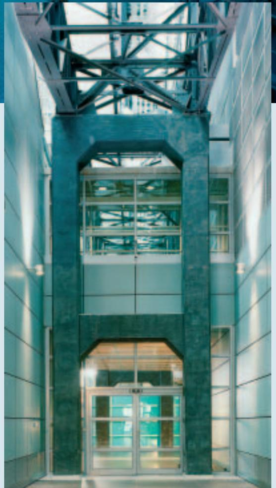
The whole roof construction rests on imposing reinforced concrete pillars. In order to provide a view of the successive pillars in the various fire lobbies, the dividing walls were also constructed in accordance to the 30-minute integrity standard with six-millimeter thick "Pyran S" in a Schueco profile system.
