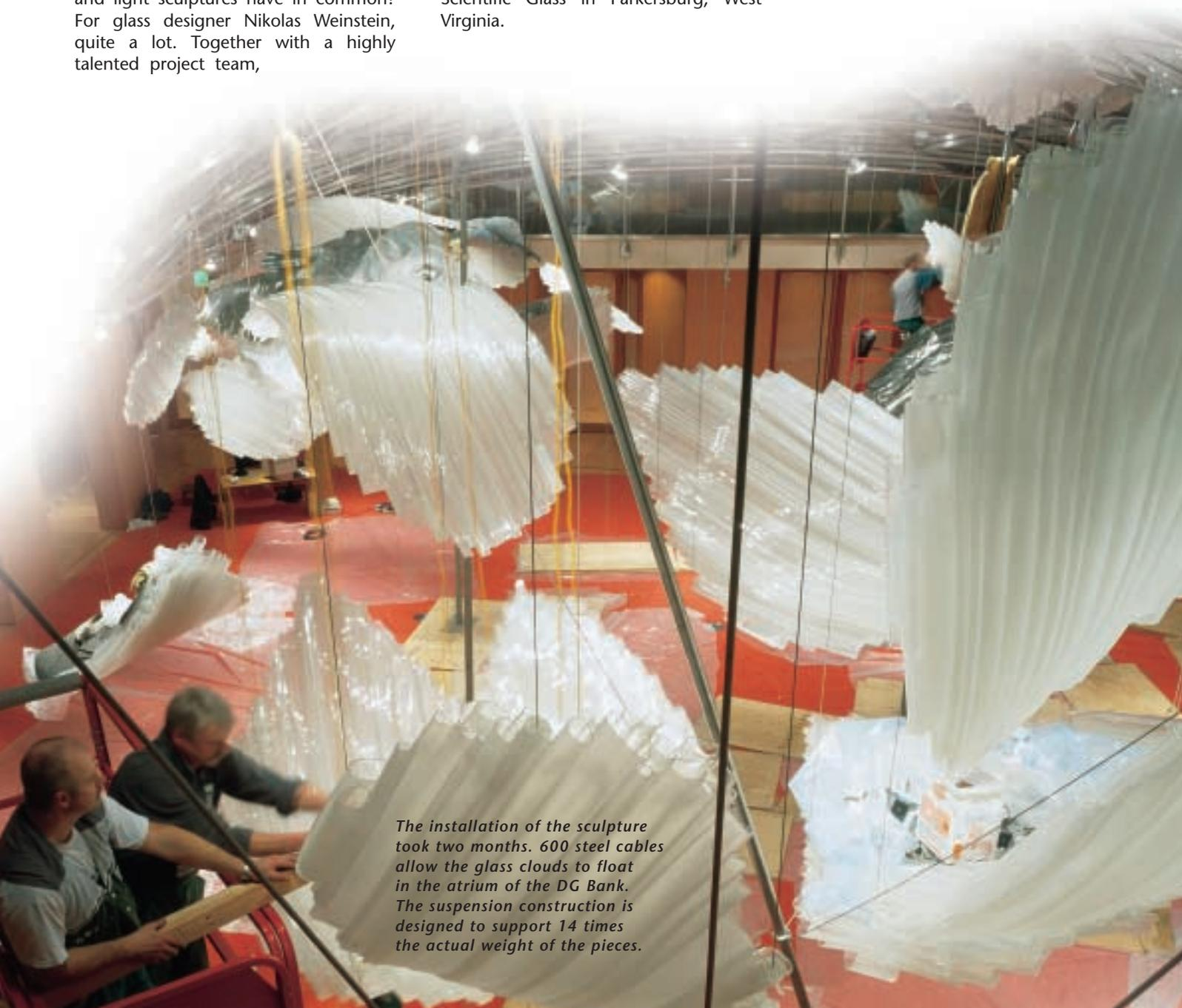
*The installation of the sculpture took two months. 600 steel cables allow the glass clouds to float in the atrium of the DG Bank. The suspension construction is designed to support 14 times the actual weight of the pieces.*
