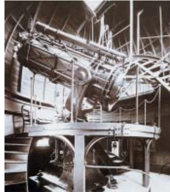
The first mirror telescope of the University of Heidelberg began operations on the Königsstuhl in 1906. The mirror substrate from SCHOTT measured 720 mm.
