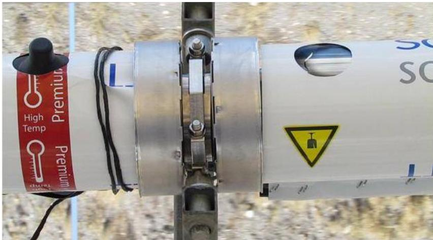
Fig. 4. Field installation of SCHOTT's 4<sup>th</sup> Generation receiver.
