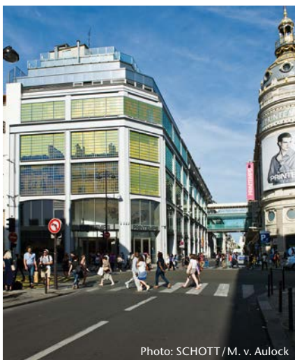
Photo: SCHOTT / M. v. Aulock
