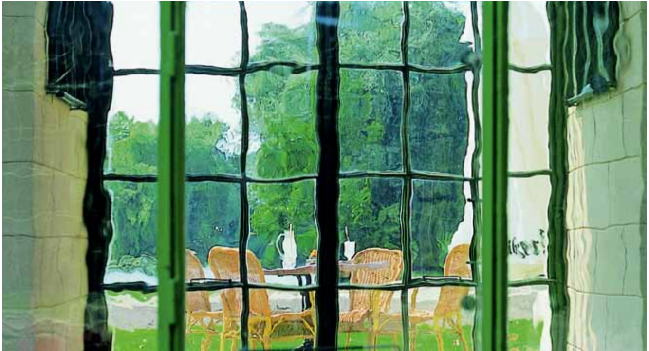
Orangerie at Schloss Schwerin (Germany): The historical character of the windows was preserved with RESTOVER® glass for restoration.
