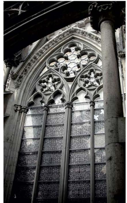
The Cologne Cathedral received its first protective glazing in 1980, a solution using monolithic panes. However, the laminated safety float glass used has the disadvantage of constant reflection. Since 2003, an anti-reflective glass has been used as protective glazing for the medieval choir windows. Reflections from the sky and neighboring buildings as well as shadows from the buttresses, which vary according to the position of the sun, needed to be reduced as much as possible.
