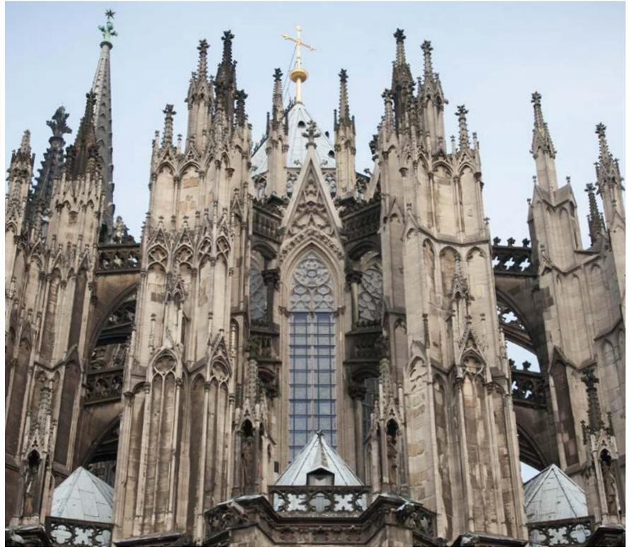
square at the Cologne Cathedral using glass samples with anti-reflective and optical interference properties from various manufacturers, had noticeably high degrees of reflection and intense color reflection. The anti-reflective system from SCHOTT minimizes these reflections and allows an almost unadulterated view of the original glazing.
