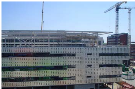
AMPPS Building under construction in Manchester
