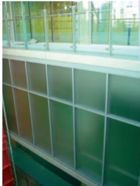
Evelina Children's Hospital, London: Sandblasted PYRAN® S offers privacy as well as reassuring safety.
