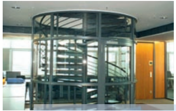
PYRAN® G curved fire resistant glazing provides both safety and aesthetic properties, as in the Fraunhofer Haus in Munich.
