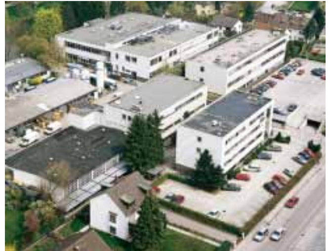
SCHOTT Electronics GmbH and SCHOTT Electronic Packaging GmbH (Plant I), Landshut, Germany
