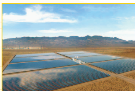
Parabolic trough power plant in Nevada (photo rendering), which is scheduled to begin providing energy to the grid in 2007
