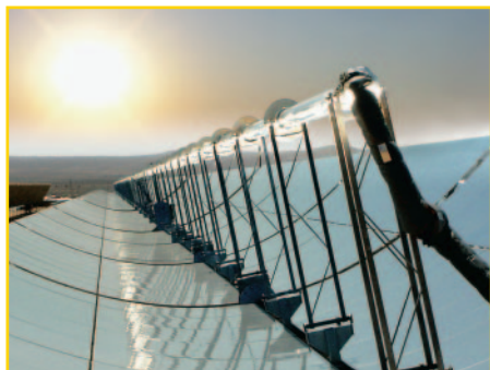
Parabolic trough with receivers
