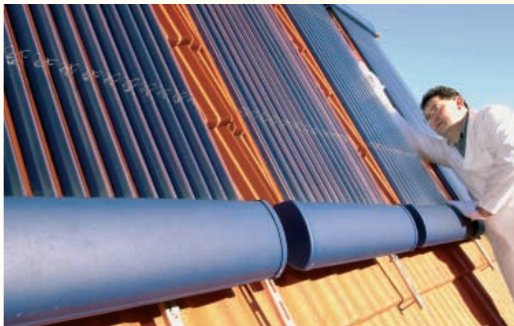
To increase energy yields, Schott-Rohrglas plans to develop improved anti-reflection coatings for tube collectors (above) and parabolic troughs (below).
