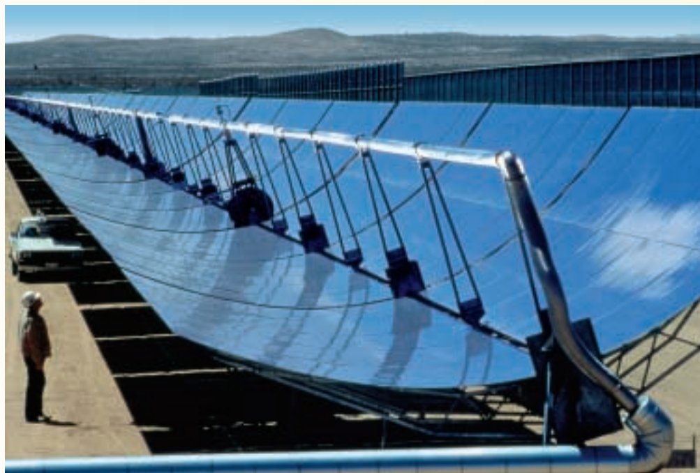
To increase energy yields, Schott-Rohrglas plans to develop improved anti-reflection coatings for tube collectors (above) and parabolic troughs (below).
