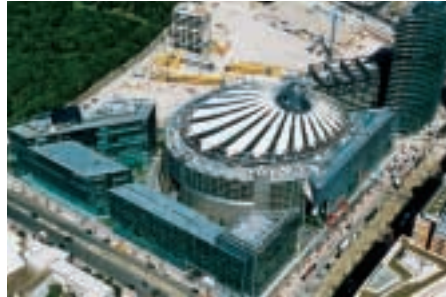
On Potsdamer Platz in Berlin, Sony has built a futuristic entertainment complex with offices, shops and apartments. The 26,500 square meter center cost 750 million euro.
