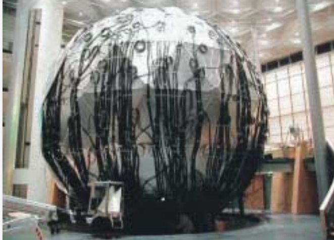
Intricate inner workings: the individual light panels of the illuminated "Kugelhaus" are supplied with light from 20 kilometers of light conducting cables.
