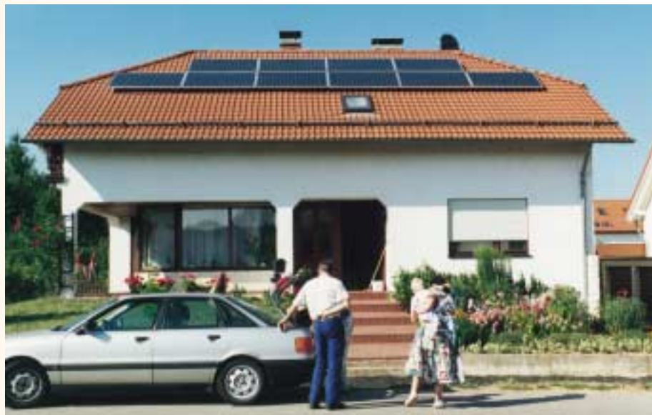
A photovoltaic unit on the roof of a single-family house: the most solar energy is produced when the modules face south and are installed at an inclination angle of 30°.
