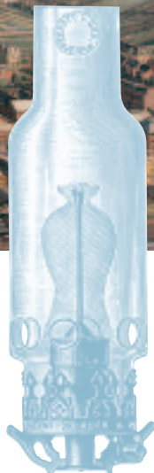
With the mass production of heat and thermal shock resistant cylinders for the Auer incandescent gas lamp, the Glass Technology Laboratory grew into an industrial concern.
