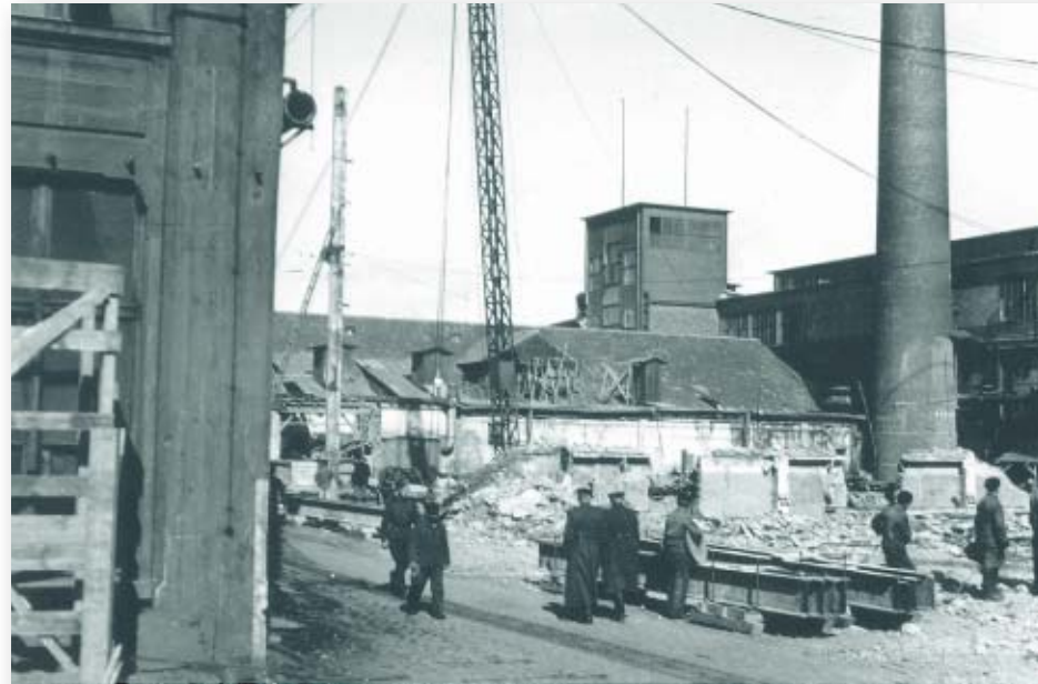
Soviet soldiers completely dismantled the production facilities, even some of the buildings.
