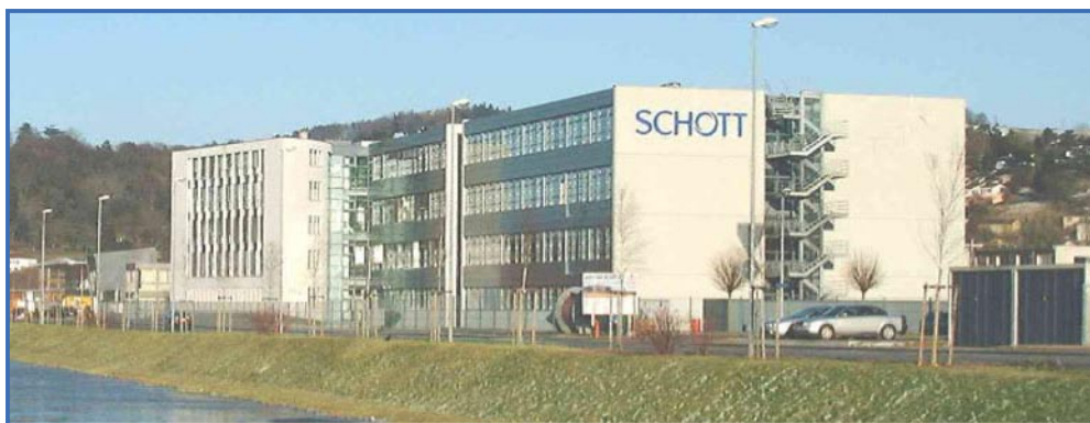
The building in Yverdon
